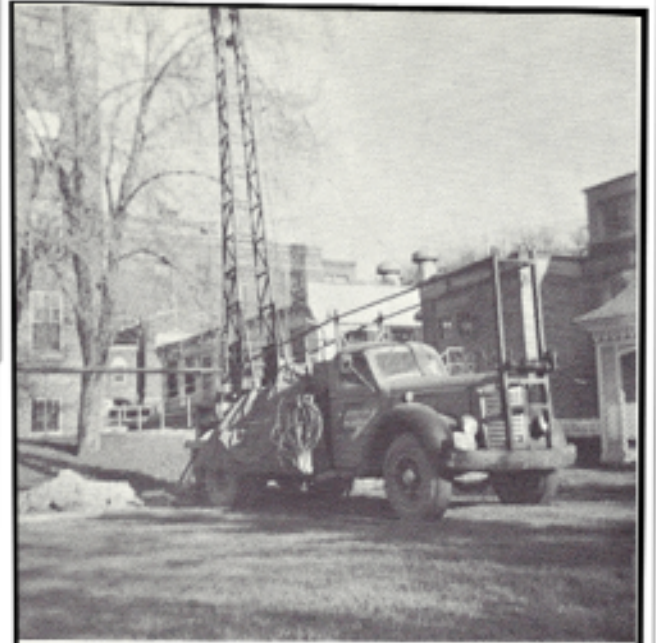
THE FIRST PIECE OF EQUIPMENT THAT CAME TO TEAR DOWN STAFF AND MARYGROVE.
